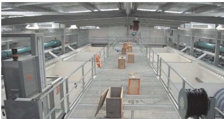
**Submerged microfiltration system similar to the OCWD, Water Factory 21 California system to treat 325,000 m<sup>3</sup>/day secondary sewage pre RO for saline ingress control and indirect potable reuse. Decision based on 25 years of RO operating experience and extensive pilot studies repurifying wastewater.**
