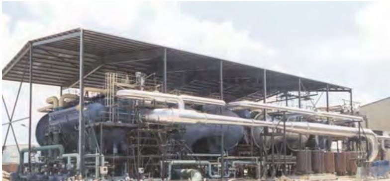
*The Curacao plant uses a thermo-compression distillation (MED) to produce potable water from seawater.*
