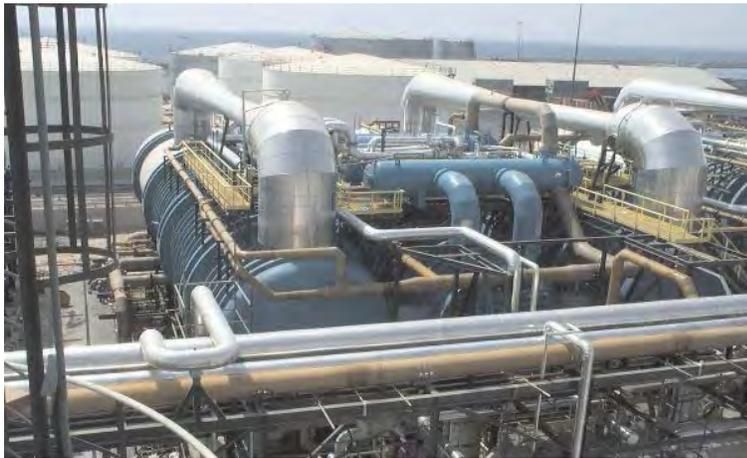
**High efficiency MED installation in UAE.**
