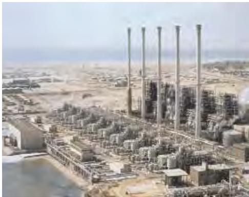
*Al Khobar Phase II MSF coupled to power plant in Saudi Arabia. 1979, 267,000 m3/d*
